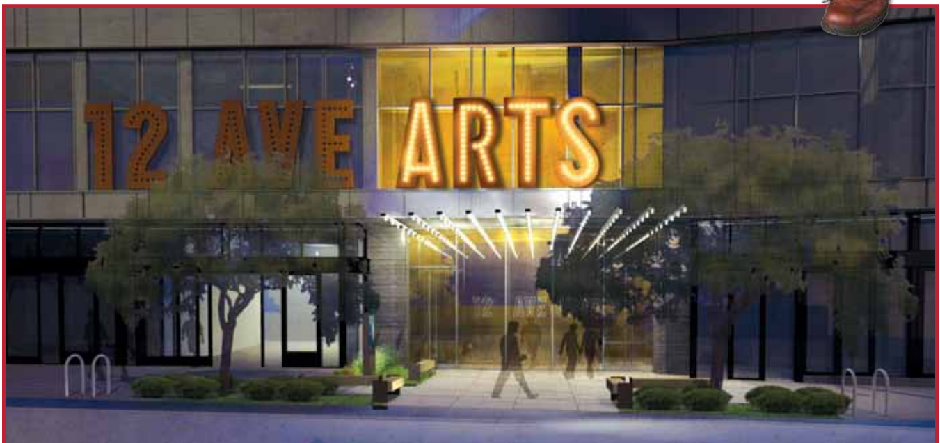
12 Ave Arts is now under construction.
