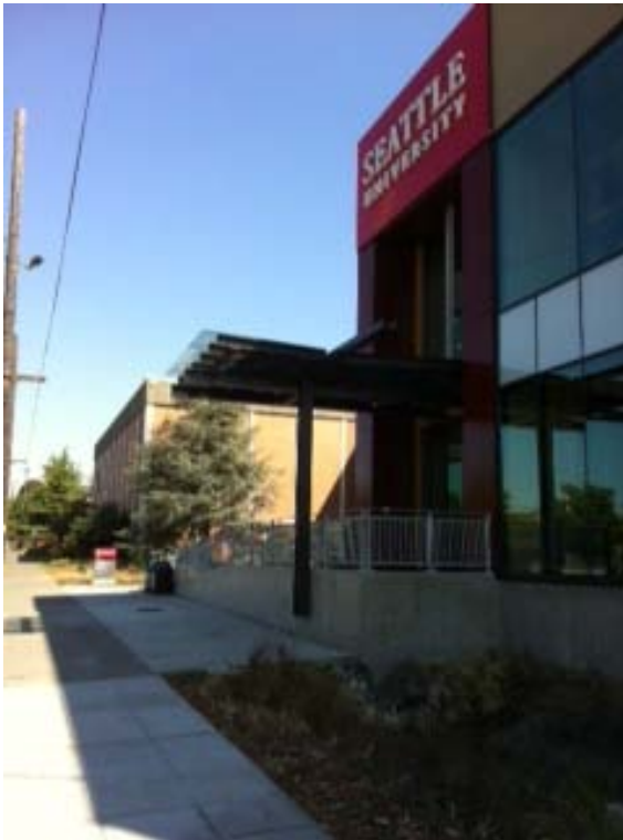
New entrance to the Connolly Complex
