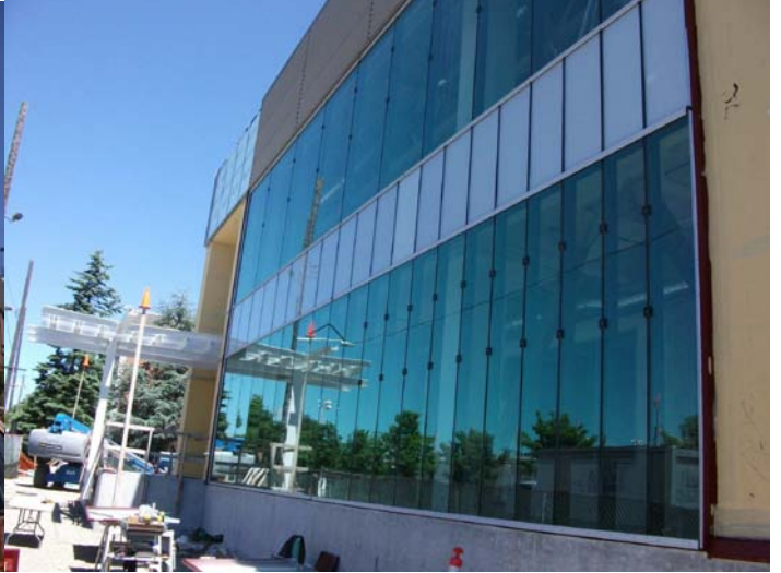
Completion of the curtain wall system
