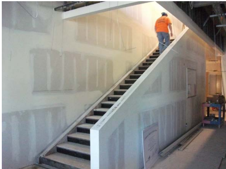
Completion of tape, mud, and sand in preparation for painting
