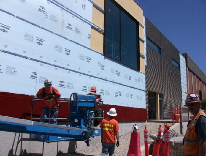
Installation of colored metal panels
