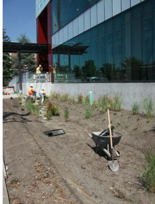
Installation of Landscaping at Rain Garden Swale
