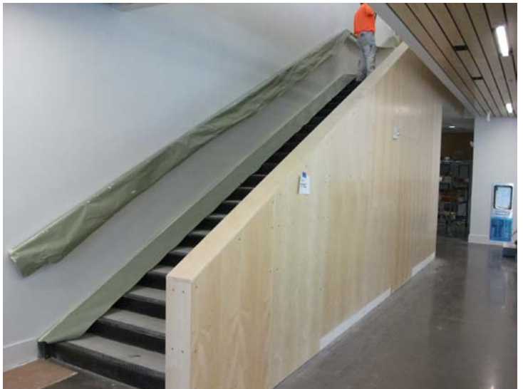
Entry Staircase Plywood
